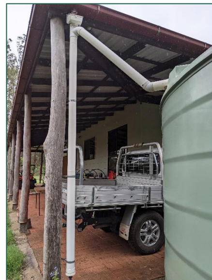
A first flush system for rainwater tanks. Credit: Ray/Wendy Benfer.
